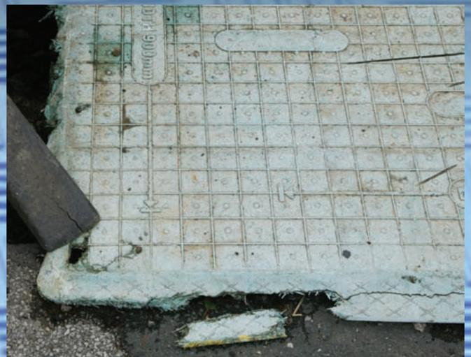
Trench-Guards do not splinter on the edges (unlike fibreglass or plywood).
