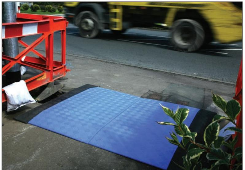
Trench-Guards provide ideal pavement crossings for vehicles and pedestrians during utility works.
